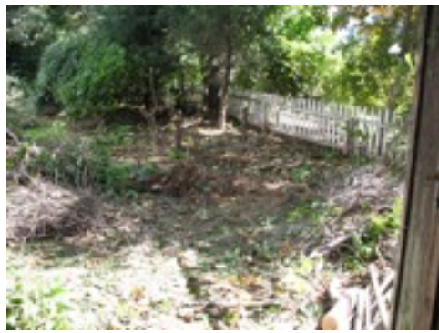
Clearing the yard
