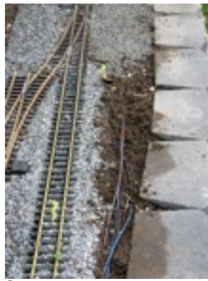
DCC wiring underground
