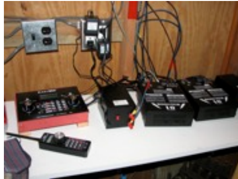
DCC controls in shed (Easy DCC by CVP)
