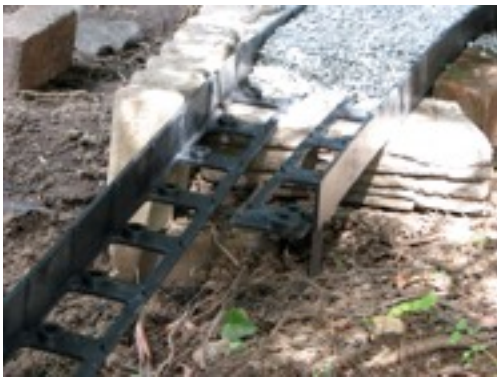
Start of trestle
