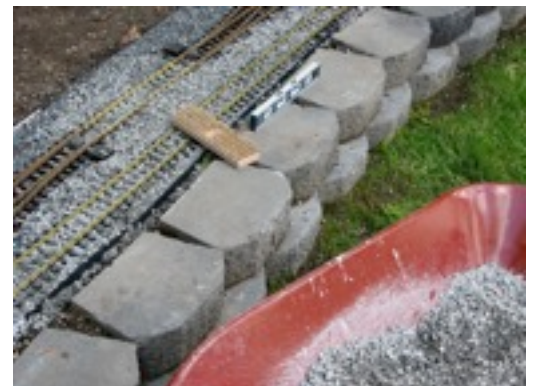
Track leveled with 1/8" bluestone
