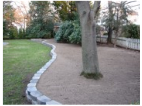
ground raised and leveled
