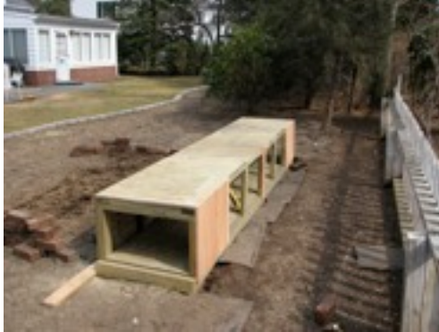
backside access to tunnel
